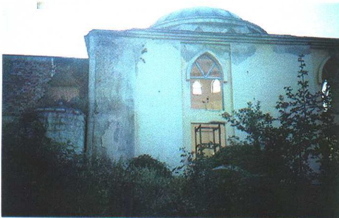
photo from: Islamic Community of Dobož - side view; stump of toppled minaret and hole in wall of mosque visible at left
