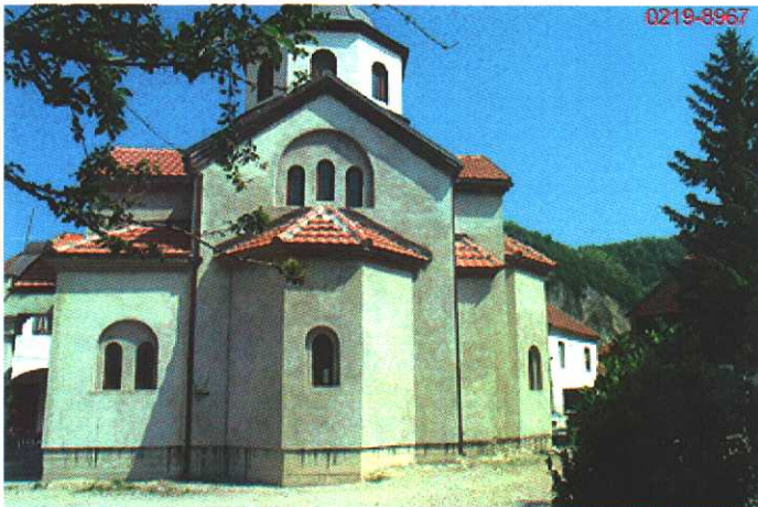
photo from: ICTY (05/2002) - new Serbian Orthodox Church built on site of destroyed Divic Mosque
